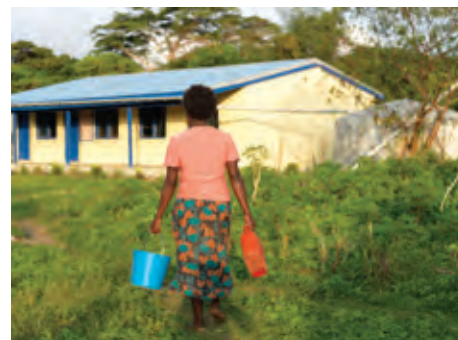
Since the construction of Napil Rural Training Centre, collecting water has been much easier for Rose (Vanuatu)
