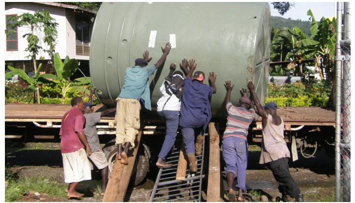
The Bougainville team load a truck with water tanks and materials ready to deliver water systems to rural communities.
