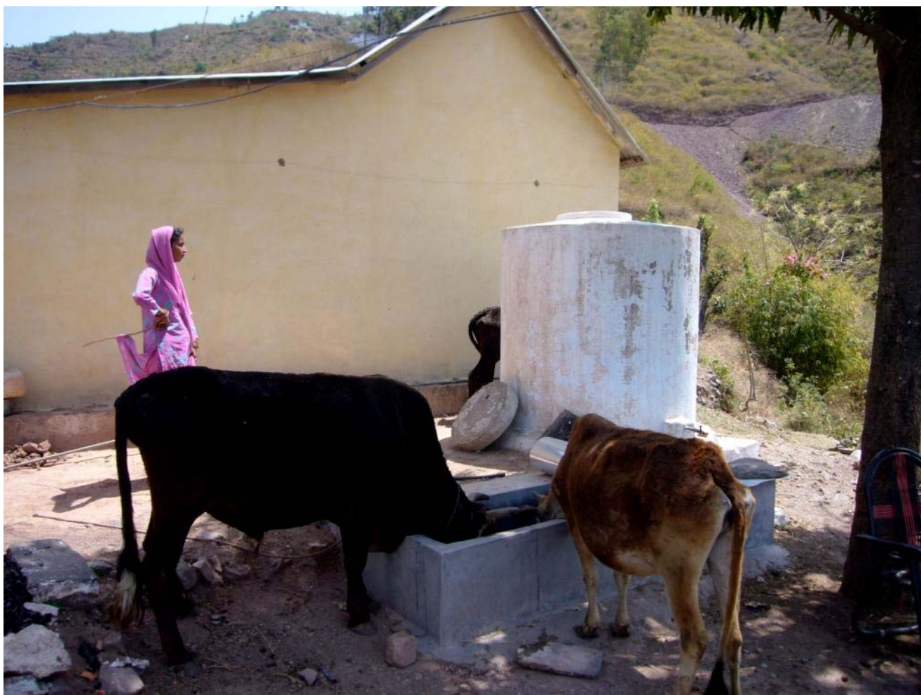
The provision of ferro-cement tanks has provided an alternative safe water supply for households during the dry season. By providing separate drinking supply for animals, water supply is further protected from contamination.
